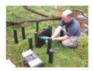
Drill and screw the top row first, locating the planks 10mm down from the top of the posts. This is to make a gap which will create a little airflow, reducing condensation forming inside the holt. Slide the lower planks onto the upper ones locking them using the tongue & groove slots and screw them in. Any gaps at the bottom can now be made up with soil. IT IS IMPORTANT TO FOLLOW THE PLAN EXACTLY. If the plan says that a corner lines up like this:
