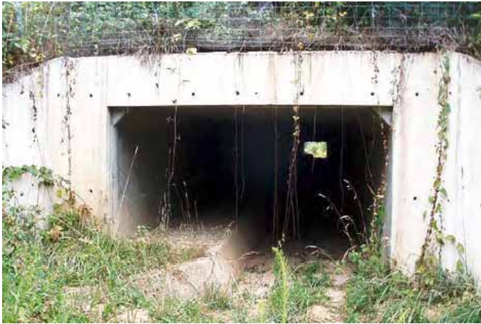
Photo 139 – Specific badger structure (approx. 3 x 2 m) – Source: V. Billon (CETE de Lyon)
