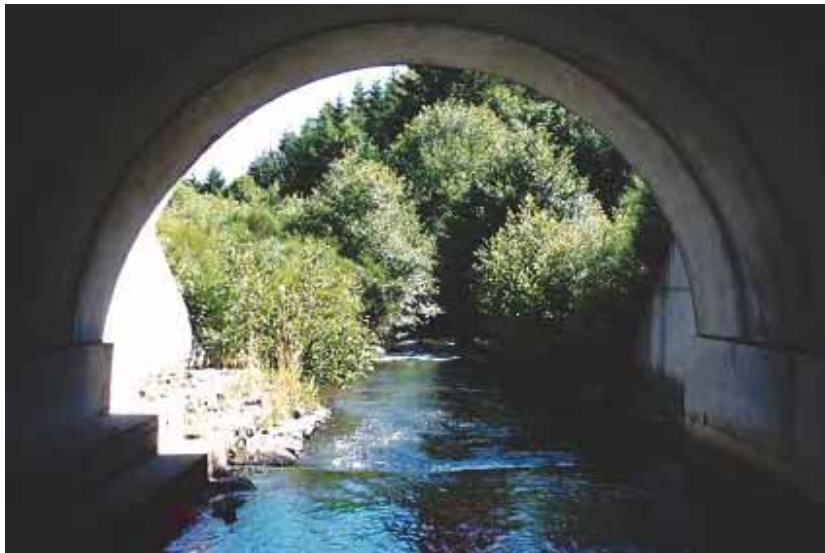
Photo 134 - RN 89 national road: otter passage on the Clidane river at the Pont du Fraisse locality (St-Jullien-Puy-Lavèze commune).
