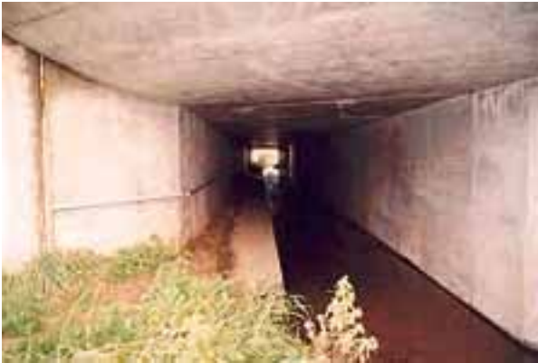
Photo 44 - A 35 motorway - DDE 67 (Bas-Rhin department): type IIIc passage. Width 3 m (incl. 1.20 m wide dry-standing), height 3 m.
