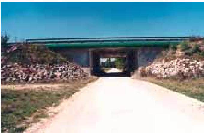
Photo 61 - A 26 motorway / SANEF (Marne department): agricultural passage (width 8 m). Clearance (perception of other side of structure) and surfacing (stabilised natural materials) favour local fauna
