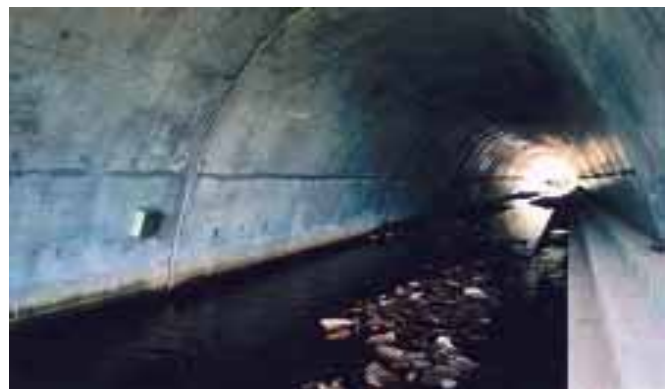
Photo 43 - A 89 motorway- Asf (Corrèze department): Dognon river crossing. Tiers (4) allow otters to cross in the dry, throughout the year, whilst remaining close to the water (on left of photo, control unit) – Source: Ch. Bouchardy
