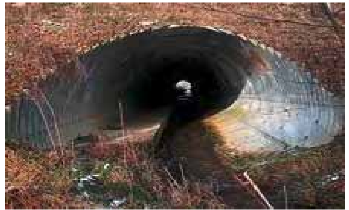
Photo 40 - Type IIIa passage: steel pipe with 1 m wide ledge
