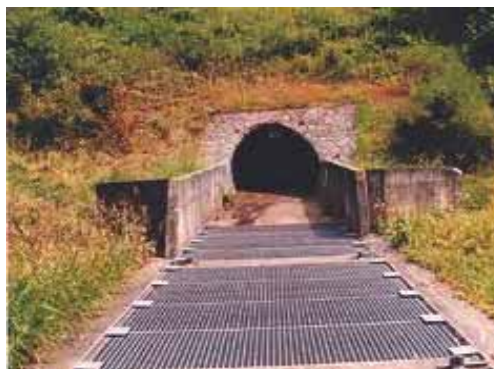
Photo 59 – Grating prevents fauna access to the passage
