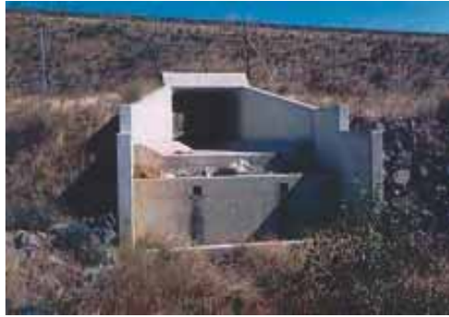
Photos 54 and 55 – Overdesigned hydraulic structure, often dry (Mediterranean regime) but unusable to fauna.
