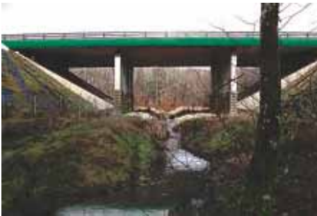
Photo 49 - A 89 motorway - ASF (Dordogne department): slab bridge crossing of "Boutouyre" stream. Deck width: 25 m.
